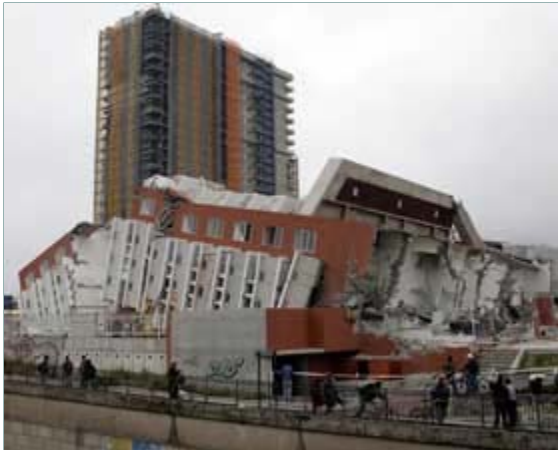
A collapsed building in the after math of the 8.8 magnitude earthquake in Chile Image from Wikipedia Commons.
